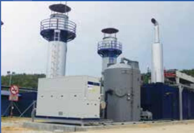
KUB-Energy landfill gas engine and gas treatment system.
