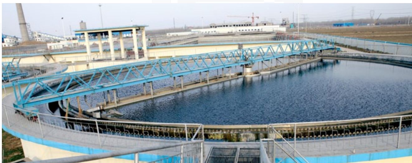
Secondary sedimentation tank of the DSG Taian Sewage Treatment Plant in the People's Republic of China.
