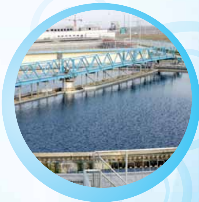
Secondary sedimentation tank - DSG Holdings' water treatment plant in Taian, People's Republic of China.
