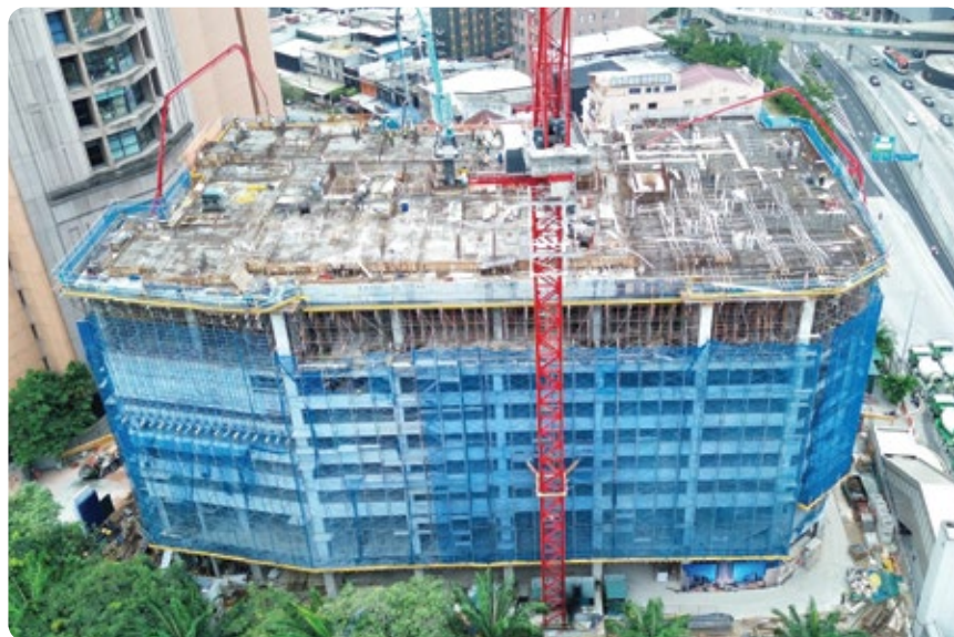
TS2 project construction progress.
