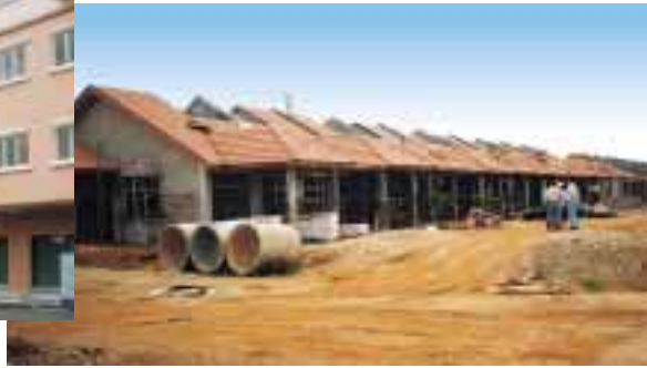
Work-in-progress of "Aspen" houses in Berjaya Industrial Park.
