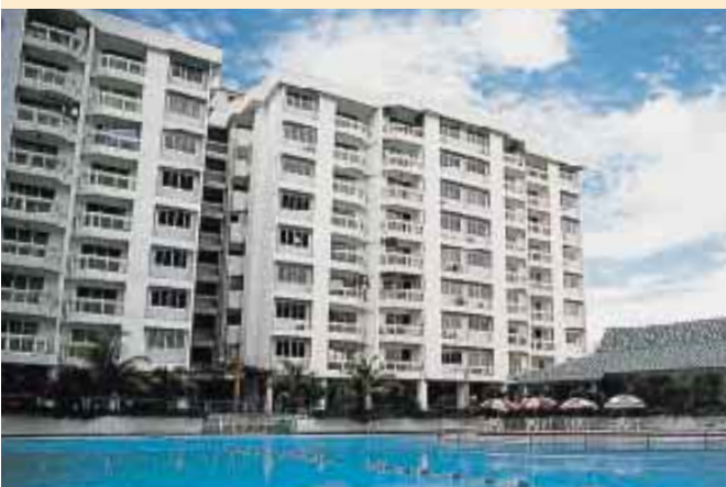
PETALING INDAH CONDOMINIUMS, KUALA LUMPUR.
