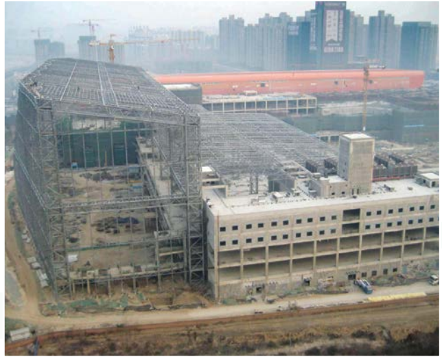
Great Mall of China - Construction in progress.
