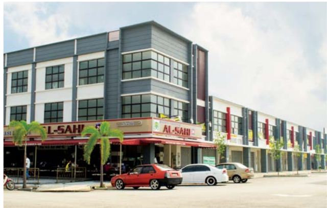
Completed Phase 2 & 3 of Trade Point, Berjaya Park, Shah Alam, Selangor.
