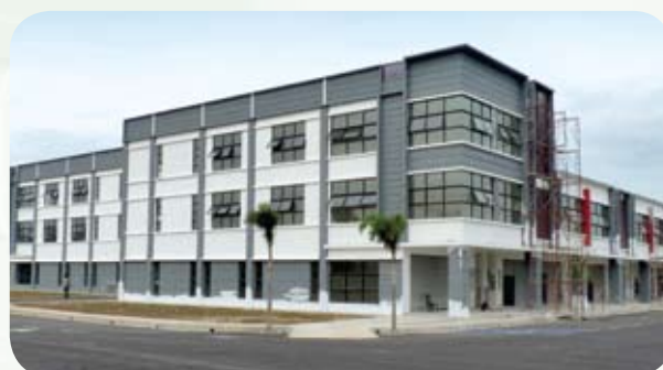
Completed Phase 1 of Trade Point, Berjaya Park, Shah Alam, Selangor.
