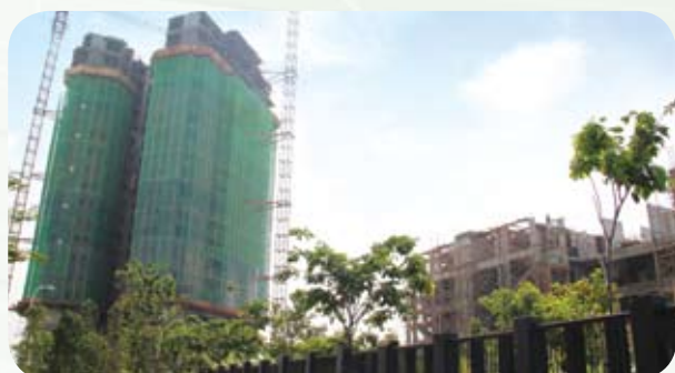
KM1 East Condominiums, Bukit Jalil, Kuala Lumpur - Construction in progress.
