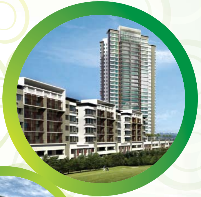
KM1 East Condominiums, Bukit Jalil, Kuala Lumpur.
