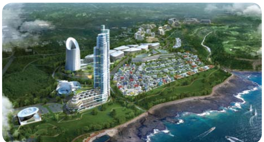
The perspective view of Berjaya Jeju Airst City, Jeju Island, South Korea.
