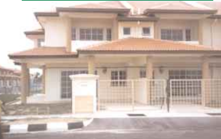
Mulberry, comprising 180 units of double storey terrace houses at Berjaya Park, Shah Alam.
